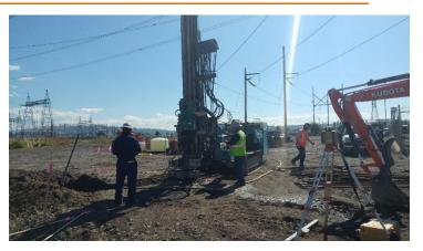
energized overhead and adjacent power lines. We began the project testing to assure we were achieving proper loads and to potentially reduce the quantity. We were able to eliminate some of the bigger bars, proof test fewer in the end saving both the contractor and owner money.
